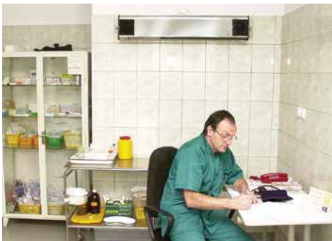
One of the important advantages of flow UV-C germicidal lamps with forced air flow is a possibility of their use in the presence of personell and patients (permanent disinfection of the air)
